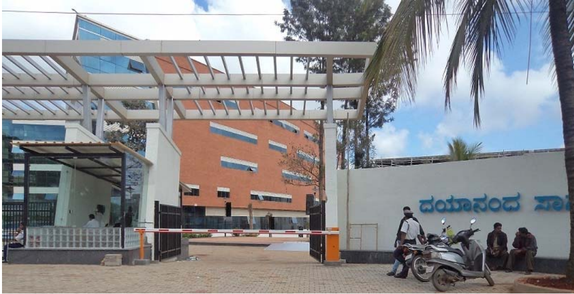
PROJECT: DAYANAND SAGAR KAKAKPURA ROAD.
