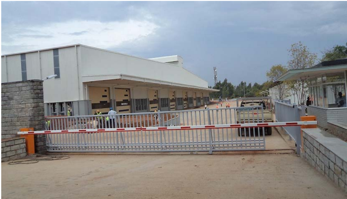
PROJECT: OTIS ELEVATORS JIGNI BANAGLORE
